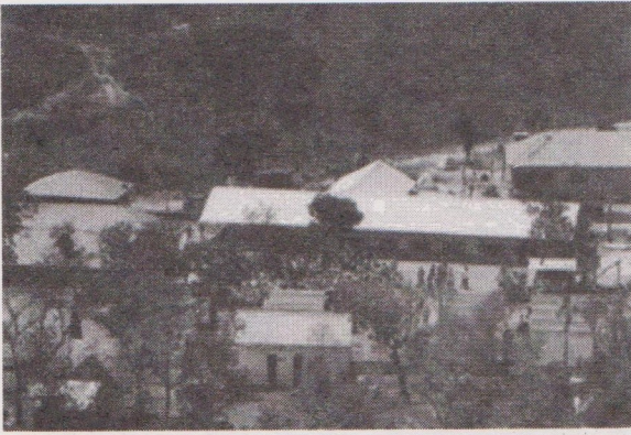
The Project Portal compound on the "farm" of Urandir.
